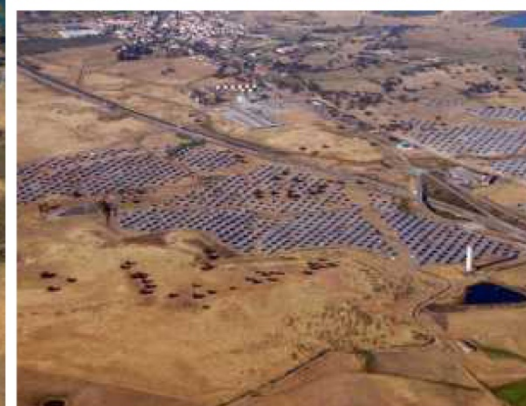
Almaraz, Spain Total: 20MWp (6 MWp of arinna)
