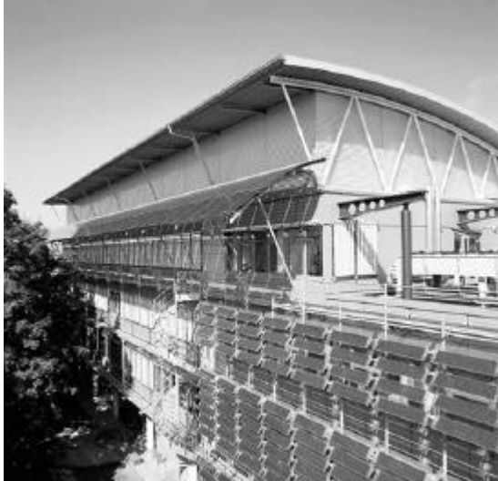
Fig. 6: Façade of the Clinical Molecular Biological Research Centre with two BIPV solutions
