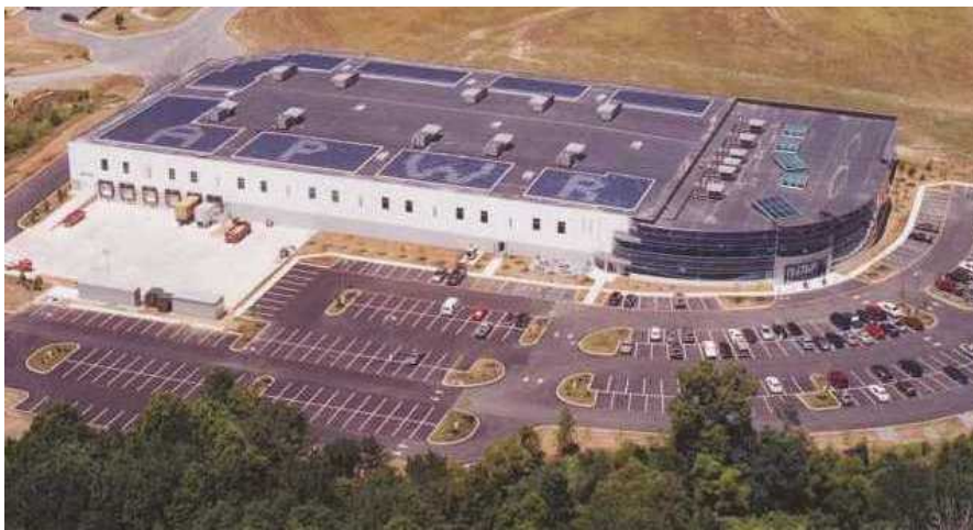
Fig. 6: 310kW p BIPV façade and rooftop system
