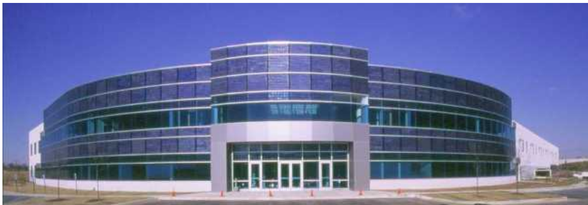
Fig. 3: AstroPower, Inc. headquarters BIPV façade in Newark, Delaware, USA
