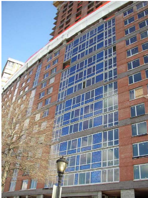
Fig 2: Solair – BIPV façade during construction
