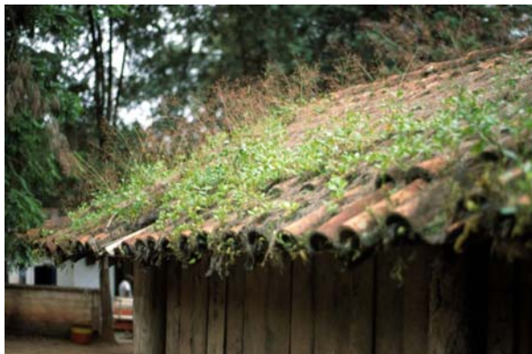
Fig. 1: A spontaneous green roof on a small house in Minas Gerais, Brazil.
