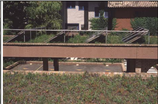
Fig. 4: Florianopolis: Extensive green roof construction with solar heating systems over parking lots. Green roof with Delosperma othona .
