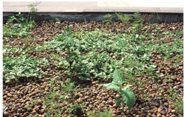
Fig. 2: Extensive green roof on MAM Building, Rio de Janeiro, Brazil
