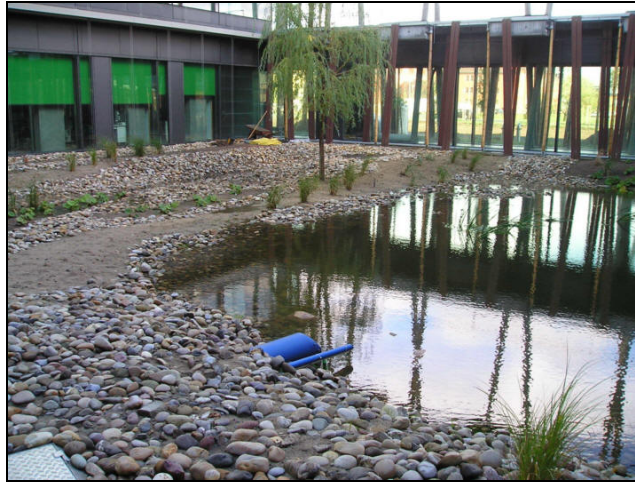
Fig. 12: Constructed lake with natural surface infiltration
