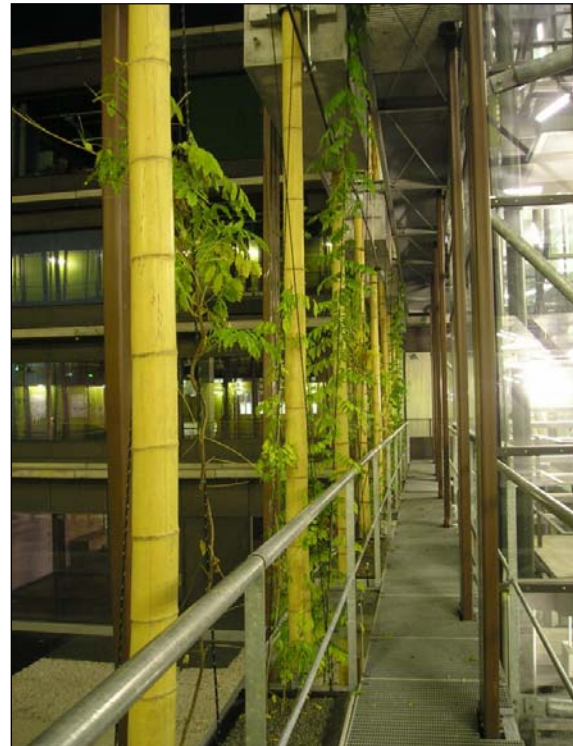
Fig. 10 and 11: Climbing plants provide shade and cooling by evapotranspiration (left: in construction 10/2003)
