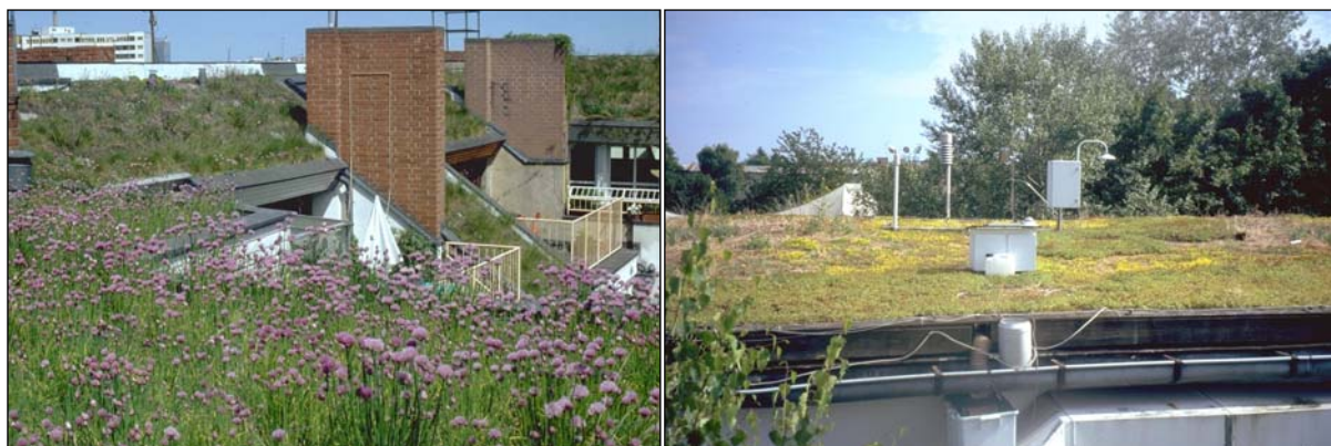
Fig. 6 (left): In 1984 greened roof in Berlin's city center (Paul Lincke Ufer 44, Berlin Kreuzberg)
