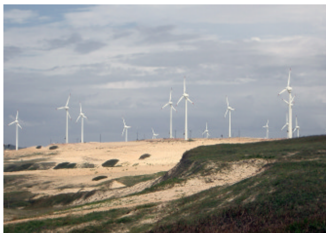
Fig. 1. Brazil's largest wind park: Prainha (30 km from Fortaleza, in the Northeast of Brazil) with 20 wind turbines of 500 kW each, representing about 40% of the country's wind power capacity presently installed.
