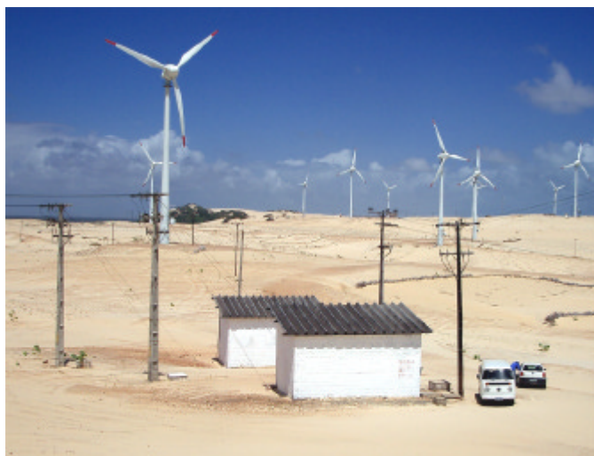
Fig. 6. Grid connection points (2 x 5 MW, in the huts) to the public grid of COELCE (to the left) at the Prainha wind park (from the right).
