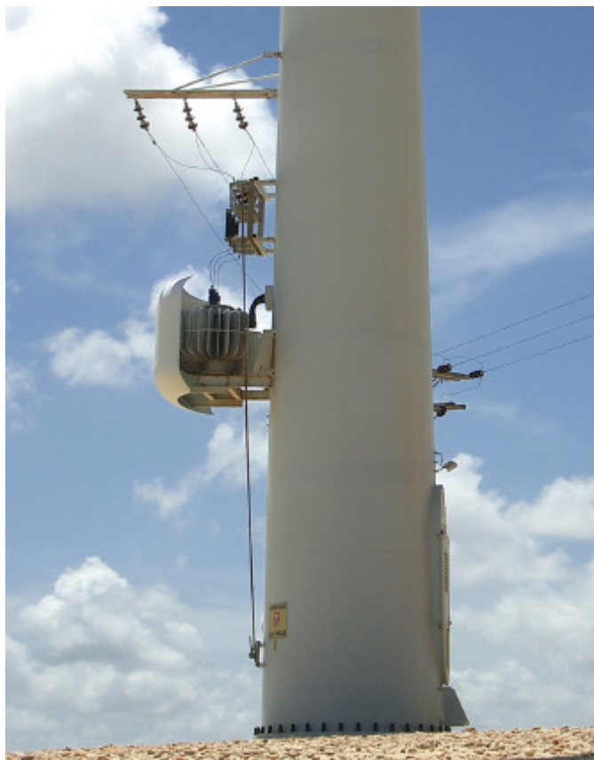
Fig. 5. A 500 kW transformer (380 V to 13.8 kV) attached to a single E 40 wind power converter.
