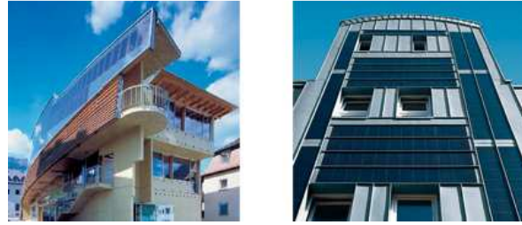
Illustration 2: Photovoltaic facade of a University building in Germany (left) [FHS Siblik] and a redeveloped residential building in Germany (right) [Rheinzink].
