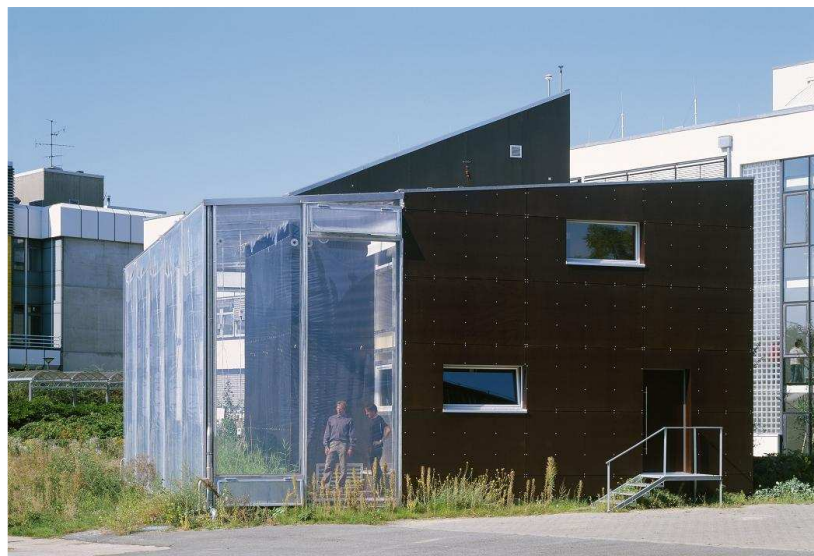
Figure 1: Demonstration building with integrated humid air solar collector system at the site of Technische Universitaet Berlin, Chair Building Technology and Design.
